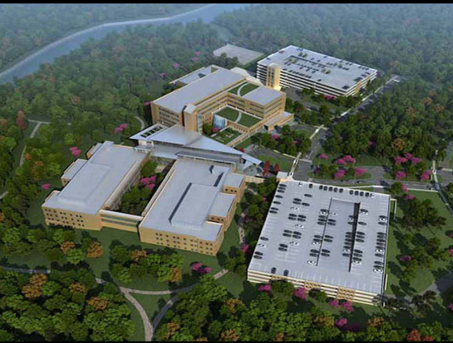
Fort Benning Hospital
